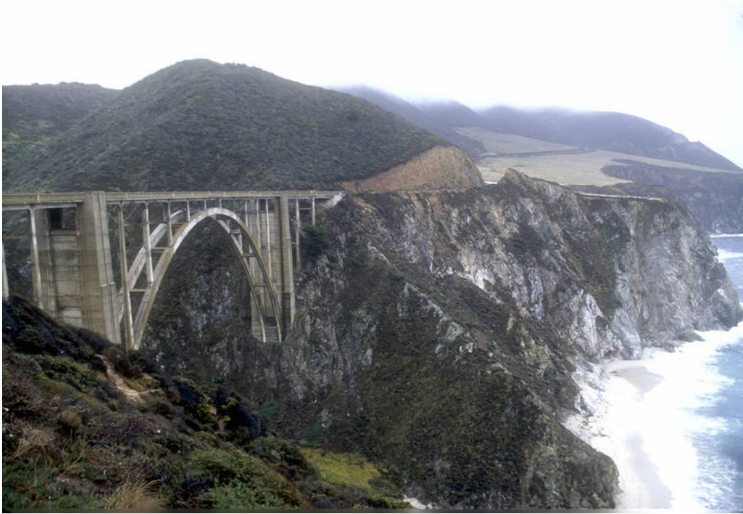
Old concrete arch bridge on California Highway 1
