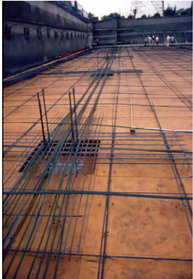
Fig. 6 – Typical Banded Tendon Layout
