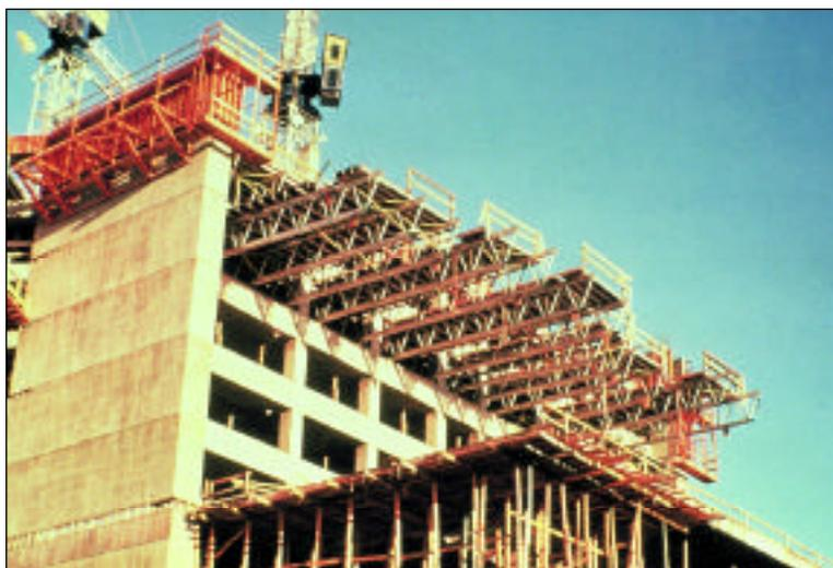
Left: Flying form being hoisted into place. Above: Flying form panels cantilevering out of multistory building, ready for flying to floor above.
