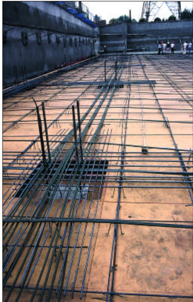
Above: Banded post-tensioned slab in a below-grade parking structure for a medical office building. Right: Looking down at banded slab construction, this photo illustrates the column reinforcing, the electrical conduit in the slab, and the pour strip between the slab and the wall to mitigate shortening and permit below-grade tendon stressing.
