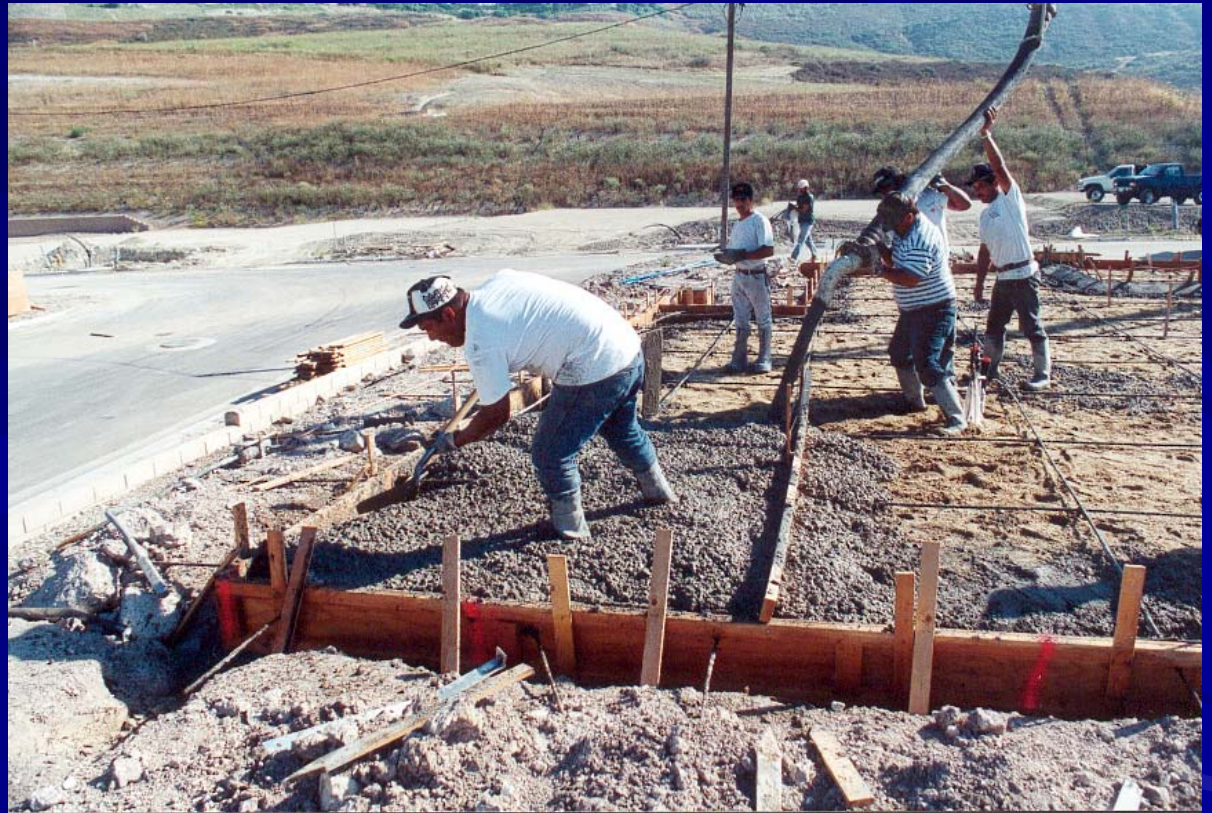
Concrete being placed in typical residential slab and footings.
