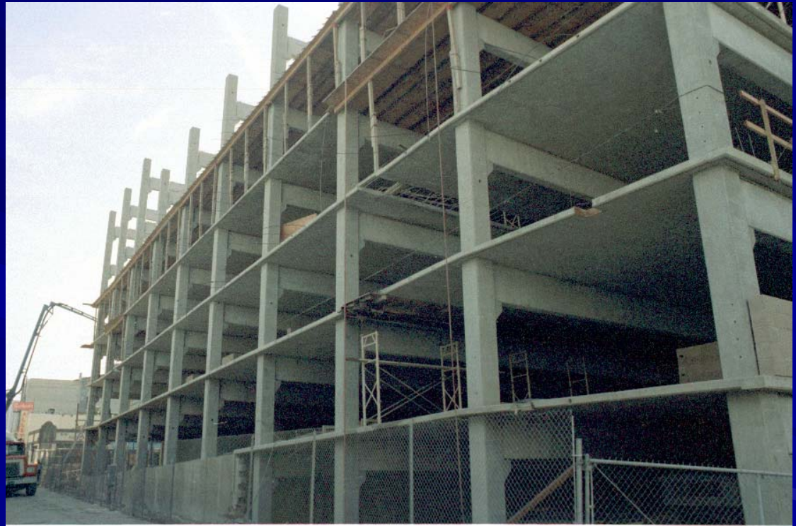
Parking Structure, Bakersfield
