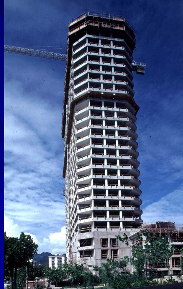
Multistory reinforced concrete apartment building under construction in Honolulu.
