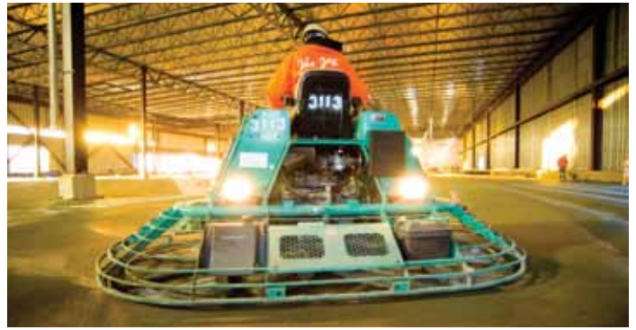
A ride on trowel levels ELEMIX at the River City Casino in St. Louis, MO. Courtesy of Syntheon.
