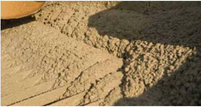
Concrete with ELEMIX being poured. Courtesy of Syntheon.
